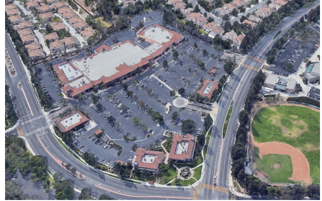
Illustrates typical multi-tenant commercial center containing anchor retail use, restaurants, and similar uses with extensive surface parking lots. (Location: Vons Center, Tierra Rejada Road and Mountain Trail Street).
