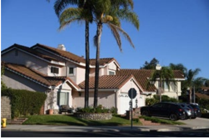
Illustrates typical single family detached units, the predominant form of existing housing in Moorpark.
