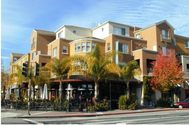
Illustrates building integrating ground level commercial and housing on upper floors, with additional height and greater building modulation to reduce sense of mass. (Location: Redwood City, CA).
