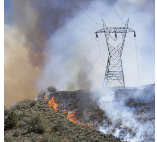
Power line tower in the wildland-urban interface fire area. Photo credit: T&D World
