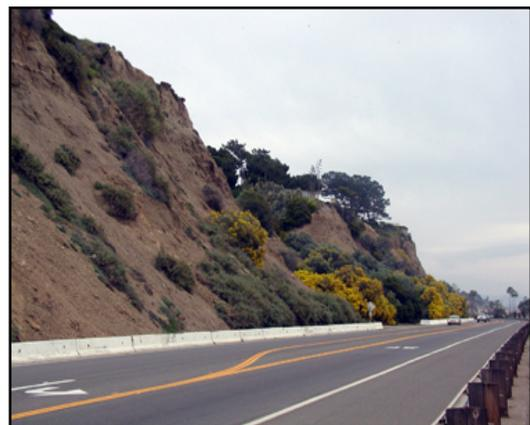
**The instability of the Capistrano Bluffs is an ongoing concern. Regulations require that development be adequately set back from bluff edges, and traffic below must be protected from potential landslides.**
