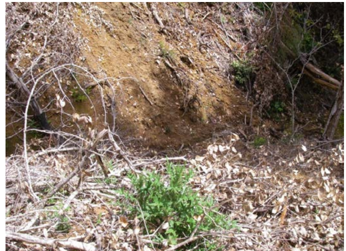
Figure 65. Abandoned crossing with significant sediment entering the channel due to slope failure (major problem), THP 1-08-176 MEN, crossing number 2.
