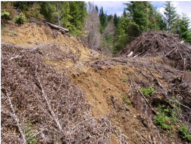
Figure 65. Abandoned crossing with significant sediment entering the channel due to slope failure (major problem), THP 1-08-176 MEN, crossing number 2.
