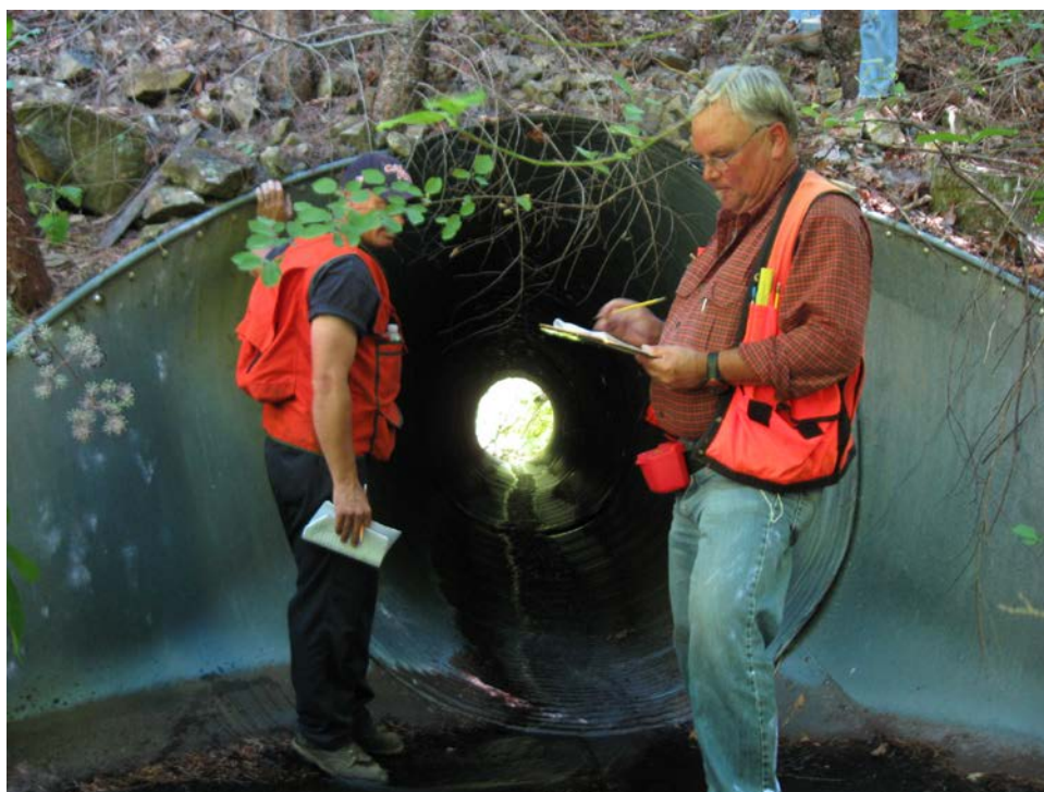
Figure 74. Clay Brandow and Gabe Schultz of CAL FIRE completing a QA/QC evaluation on a large culvert in the upper Sacramento River canyon during August 2013.
