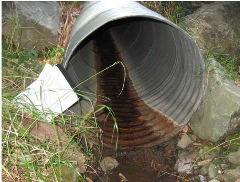
Figure 61. 36-inch galvanized steel culvert, THP 1-09-026 HUM.
