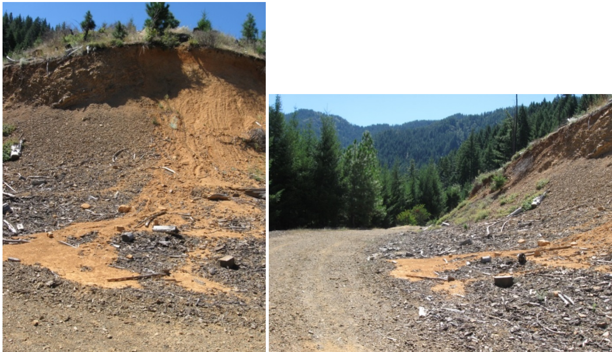
Figure 33. Example of sediment deposition onto a randomly located THP road segment in the FORPRIEM sample.
