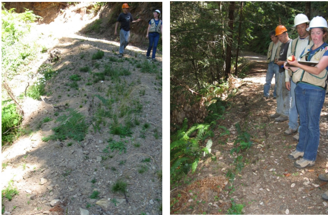
Figure 45. Some of the FORPRIEM monitoring, particularly the NTMP-NTO monitoring, was done jointly with staff from sister agencies, such as the NCRWQCB. These photos show 60 feet of road fill slope erosion on a monitored road transect (left) and tension cracks on the road surface (right).
