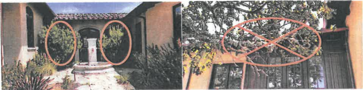
FIGURE 10 WINDOWS ARE A WEAK POINT IN STRUCTURE HARDENING; TRIM MATCHED, LARGE SHRUBS (LEFT PHOTO) 5 FEET AWAY FROM WALL AND WINDOWS. TRIM HERITAGE OAK IN COURTYARD NORTH OF HOUSE 5 FEET FROM ROOFLINE TO KEEP TREE FROM DAMAGING ROOF/GUTTER (RIGHT PHOTO ).
