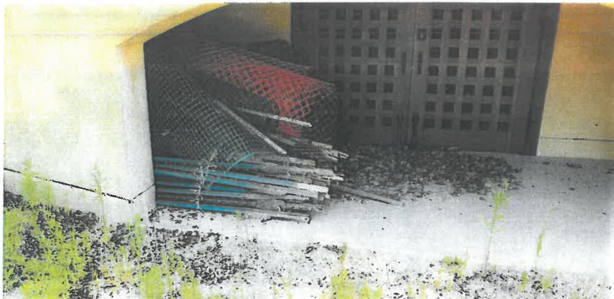
FIGURE 11 BECAUSE IT IS AN EMBER TRAP (AS EVIDENCED BY CURRENT LEAF BUILD-UP), CLEAR AWAY COMBUSTIBLE MATERIAL FROM COVERED STORAGE ENTRY.
