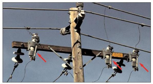
Figure 2-3 Arm Mounted Cutout with Universal Fuse
