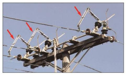
FIgure 2-38 Grasshopper Air Switch (closed position)
