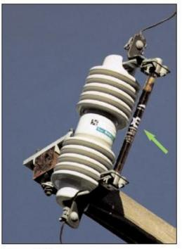
Figure 3-11 Liquid Filled Fuse
