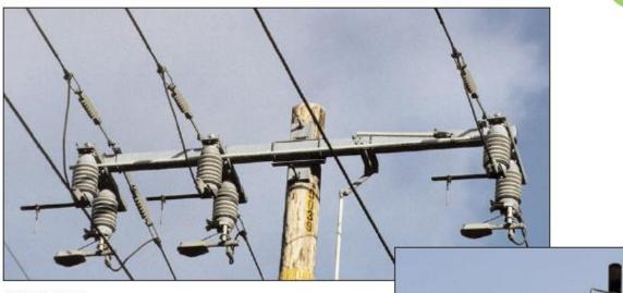
FIgure 3-24 600 Amp Underarm Sidebreak Switch (open position)
