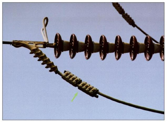
Figure 3-49 Transmission Deadend with Parallel Groove Connectors
