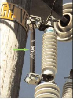
Figure 3-13 Liquid Filled Fuse
