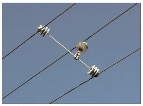
Figure 4-12 Long Span Conductor Spreader
