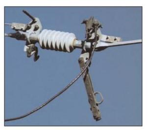
Figure 2-17 IIn-Line Disconnect (open position)
