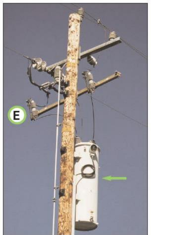
Figure 3-40 Voltage Regulator with Solid Blade Disconnects
