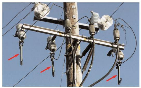
Figure 2-12 Arm Mounted Cutout with Solid Blade Disconnect (open position)
