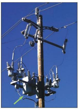
Figure 3-43 Capacitor Unit
