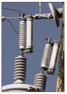
Figure 3-4 Bushing Mounted Cutout with Non-Expulsion Fuse
