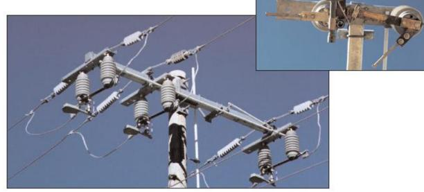
FIgure 3-27 600 Amp Underarm Sidebreak Switch (closed position))
