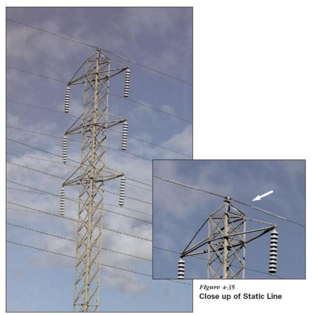
FIgure 4-34 Tangent Transmission Tower with Static Line
