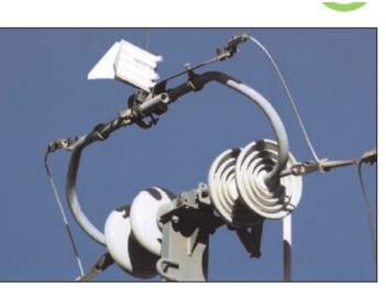
Figure 3-20 600 Amp KPF Air Switch, Triangular Construction (closed position)
