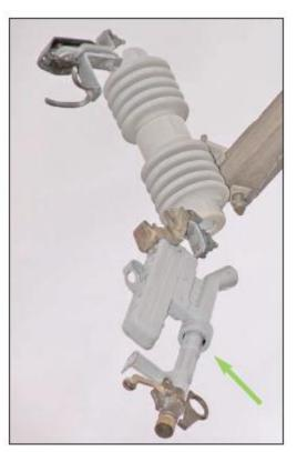
Figure 3-19 S&C Fault Tamer Fuse (Open)
