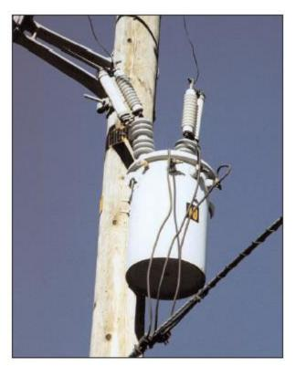
Figure 3-5 Bushing Mounted Cutout with Non-Expulsion Fuses
