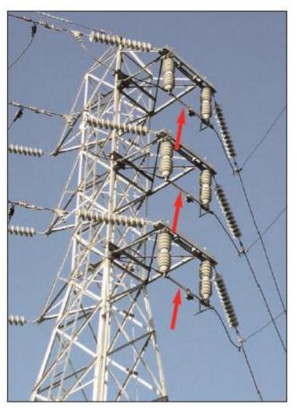
Figure 2-41 Transmission Air Switches Tower Mounted (closed position)
