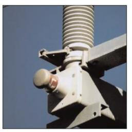
FIgure 3-35 CLosed Position Indicator Red
