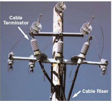
Figure 4-10 Cable Riser with Cable Terminator
