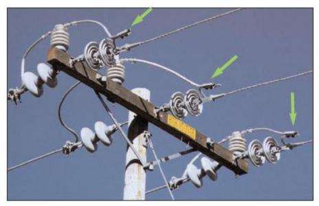
FIgure3-48 Parallel Groove Connectors on Jumpers
