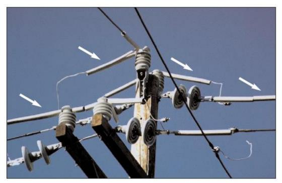
Figure 4-15 Insulated Conductor Covering
