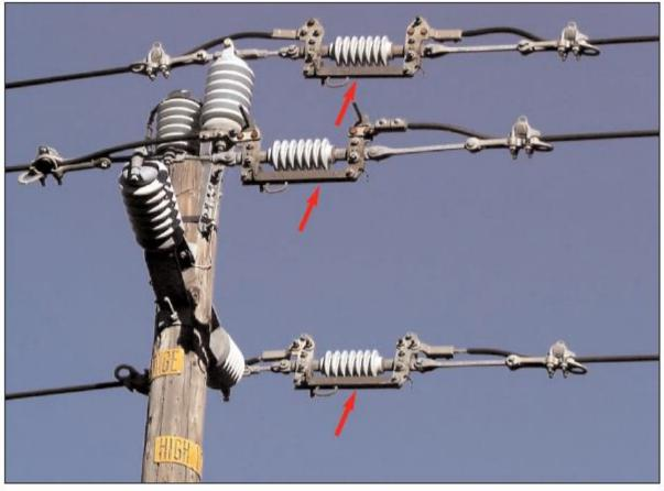
Figure 2-16 In-Line Disconnects (closed position)
