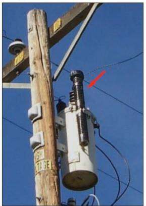
FIgure 2-28 Lightning Arrester
