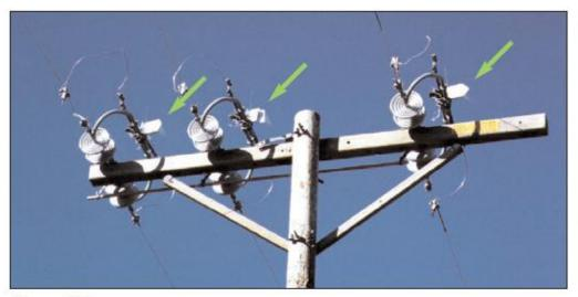
FIgure 3-22 600 Amp KPF Air Switch, Crossarm Construction (closed position) with Arcing Horns and Snuffers
