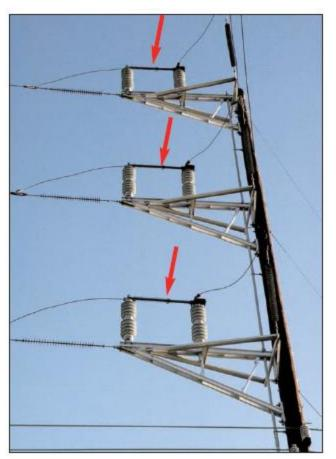
Figure 2-42 Transmission Air Switches Pole Mounted (closed position)
