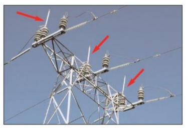
Figure 2-43 Transmission Air Switches Tower Mounted (open position)
