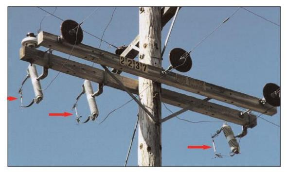
Figure 2-4 Arm Mounted Cutout with Open Link Fuse
