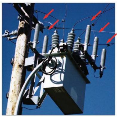
FIgure 2-20 Lightning Arrester (with Recloser)
