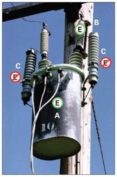
Figure 2-25 Transformer Mounted Lightning Arrester A. Conventional Transformer
