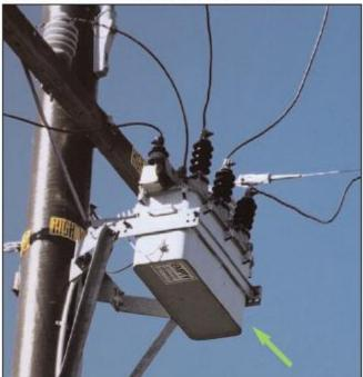
Figure 3-39 Sectionalizer Note: Only when used with Sectionalizers, Reclosers or Voltage Regulators, In-Line Disconnects and Solid Blade Disconnects are exempt.
