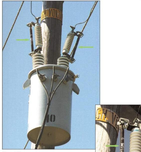
FIgure 3-12 Over head Conventional Transformer with Bushing Mounted Cutout and Liquid Filled Fuse
