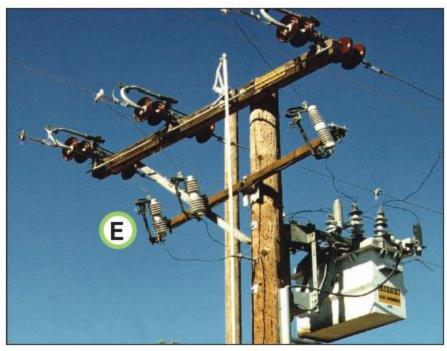
Figure 3-37 Recloser with Solid Blade Disconnects (closed position)
