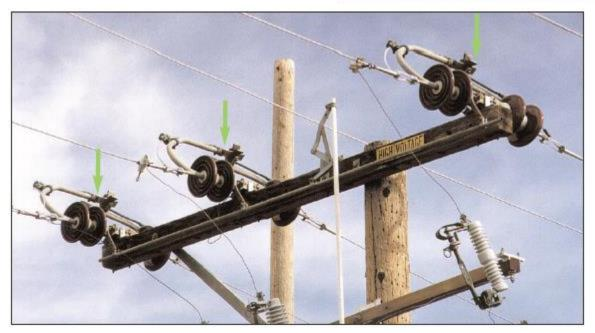
Figure 3-23 600 Amp KPF Air Switch, Crossarm Construction (closed position) without Arcing Horns or Snuffers
