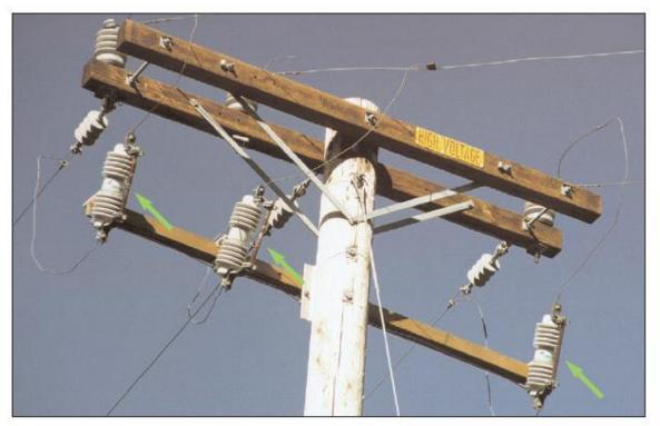
FIgure 3-10 Arm Mounted Cutout with Liquid Filled Fuse
