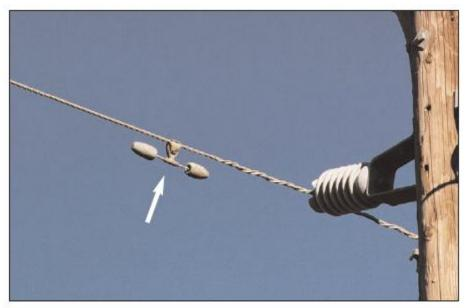
Figure 4-14 Vibration Damper
