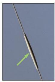
Figure 3-74 Automatic Line Splice Installed on Line
