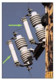
Figure 3-1 Arm Mounted Cutout with Non-Expulsion Fuse
