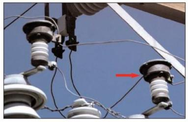
Figure 2-22 Lightning Arrester
