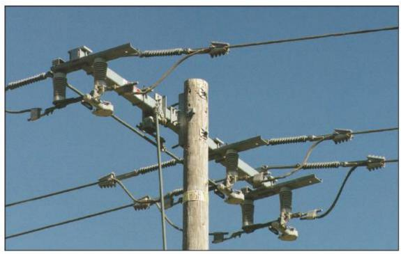
Figure 3-28 S&C 600 AmpUnderarm Side-Break Switch (closed position)
