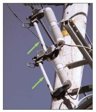
Figure 3-14 Arm Mounted Cutout with SMU-20 Fuses
