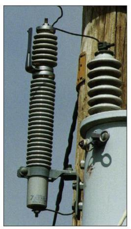
Figure 2-26 Gapped Lightning Arrester
