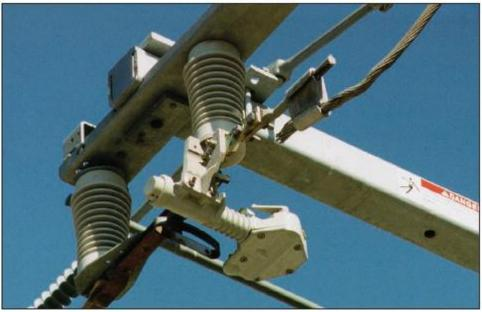
Figure 3-29 S&C 600 Amp Underarm Side-Break Switch (closed position)
