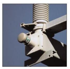
FIgure 3-34 Open Position Indicator Green Letter "O" visible
