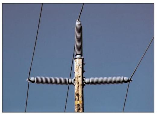
Figure 4-28 Triangular Configuration
