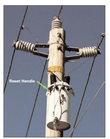
Figure 3-44 Self-Protected Transformer (no external cutouts or fuses)
