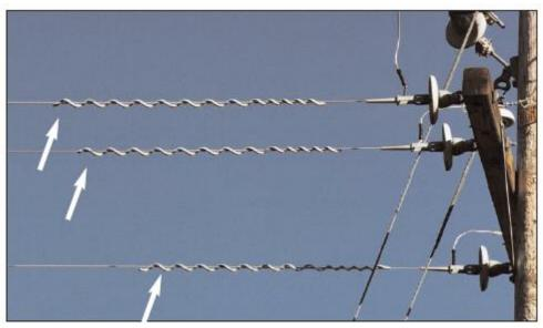
Figure 4-13 Vibration Damper
