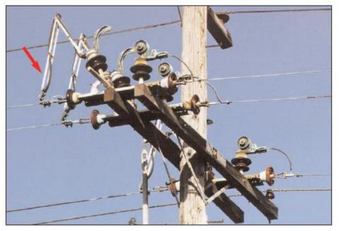
Figure 2-39 Grasshopper Air Switch (open position)
