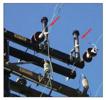
Figure 2-27 Lightning Arrester
