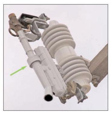
FIgure 3-18 S&C Fault Tamer Fuse (Closed)
