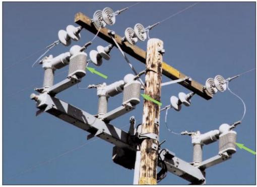
FIgure 3-33 S&C Scada-Mate Switch
