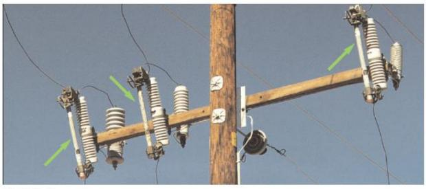
Figure 3-16 Arm Mounted Cutout with SMU-20 Fuses
