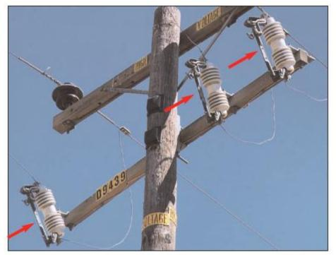
Figure 2-11 Arm Mounted Cutout with Solid Blade Disconnect (closed position)
