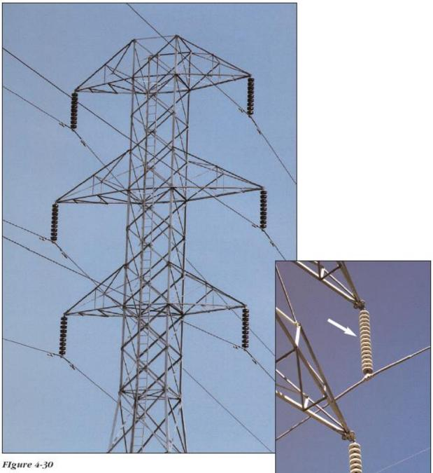
Figure 4-30 Suspension Tower
