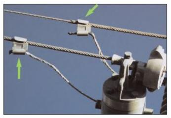
FIgure 3-60 Fired Wedge Connectors on Line
