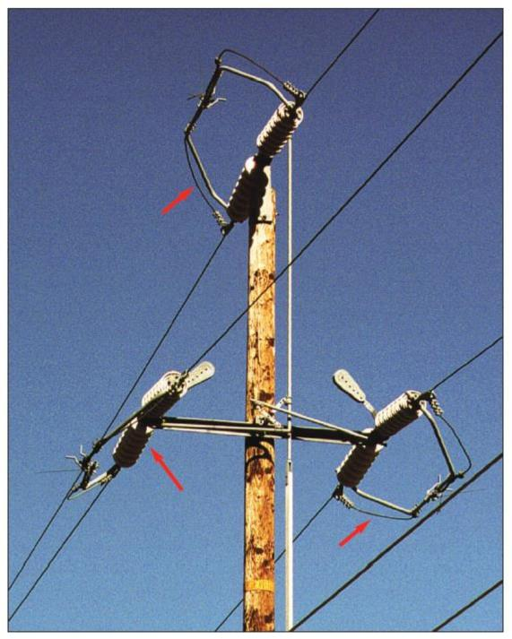
Figure 2-40 Transmission Air Switch, Pole Mounted 60kV (closed position)
