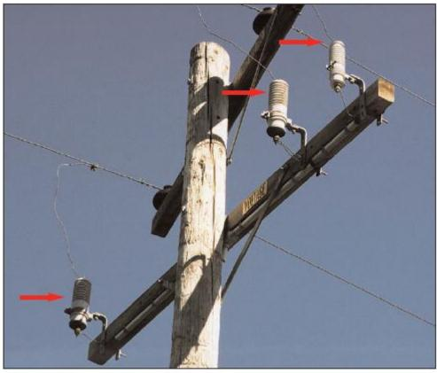
Figure 2-21 Lightning Arrester
