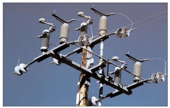
FIgure 3-30 S&C Omni-Ruptor Switch, Triangular Construction (open position)
