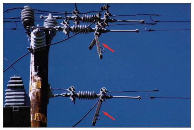
Figure 2-18 In-Line Disconnects (open position)
