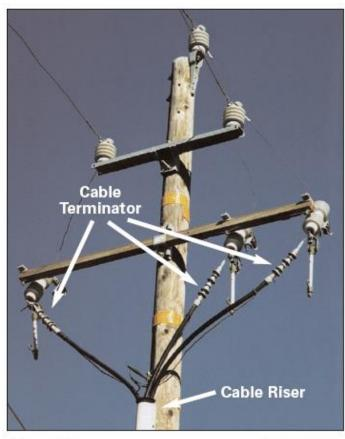
Figure 4-9 Cable Riser with Cable Terminator
