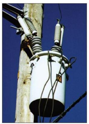
Figure 3-45 Conventional Transformer with Exempt Fuses
