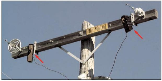
Figure 2-10 Arm Mounted Enclosed Cutout with Universal Fuses
