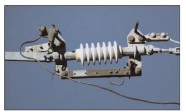
Figure 2-15 In-Line Disconnect (closed position)
