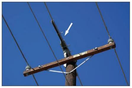
FIgure 4-22 Raptor Protector Insulator and Wire Cover
