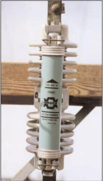
Figure 3-2 Arm Mounted Cutout with Non-Expulsion Fuse
