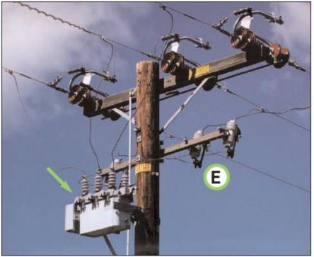
Figure 3-38 Sectionalizer with Solid Blade Disconnects
