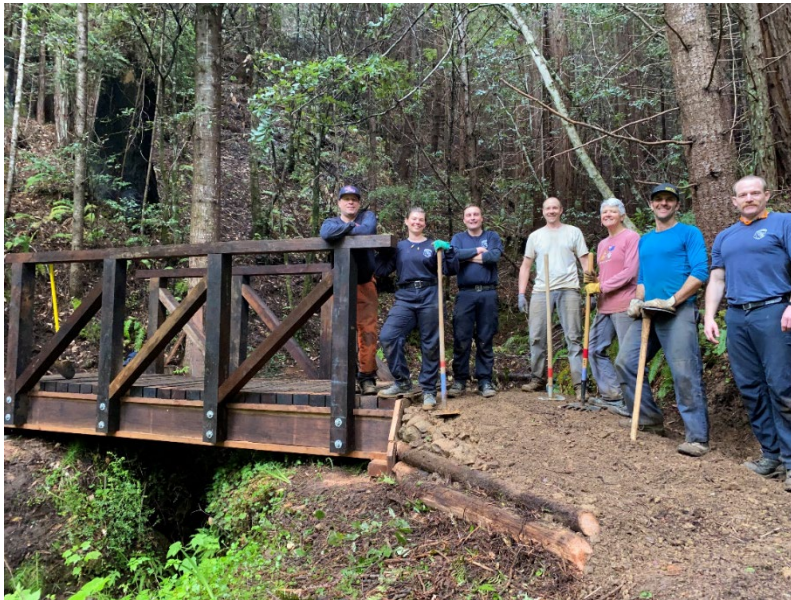
Equestrian bridge and crew on Sweetpea Trail
