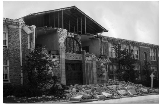
Seismic shaking primarily affects unreinforced masonry buildings, as seen here with this Long Beach middle school damaged by the 1933 Long Beach earthquake. Image from Los Angeles Times.
