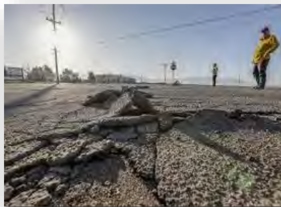
Earthquakes are high priority hazards because they are likely to happen, affect a wide area, and can be very damaging. Source Image: LA Times.
