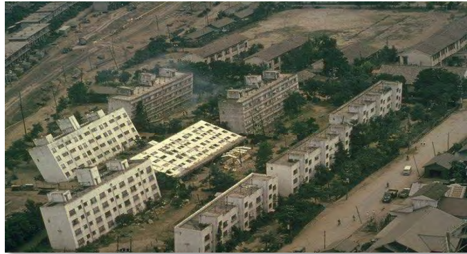
Liquefaction caused by the 1964 Niigita, Japan earthquake caused these apartment blocks to experience severe leaning. Image from the University of Washington.
