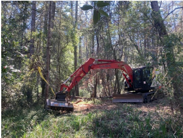
Figure 16. Example of Mechanized Equipment – Link-Belt 145 x 4 excavator with masticating head attachment
