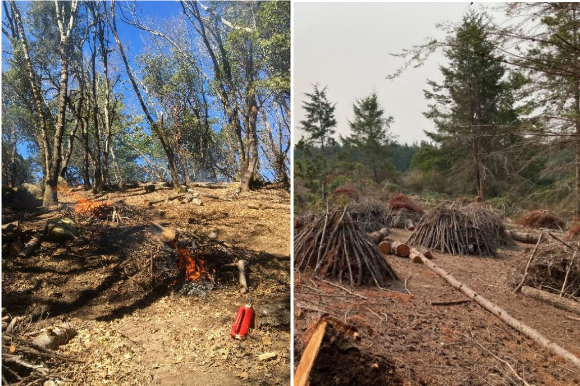
Figure 19. Pile burning operation. Castle Rock State Park (left). Quiroste Valley Cultural Preserve, Año Nuevo State Park (right)
