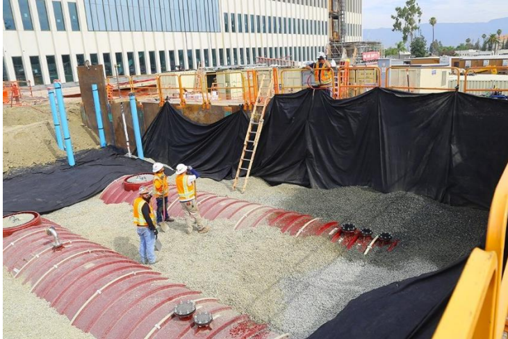
Figure 1-1. Emergency Water Tanks for Med. Center
