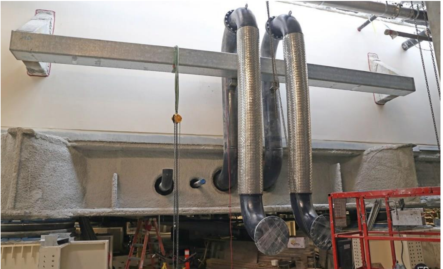
Figure 1-2: Flexible pipes in new Loma Linda University Medical Center
