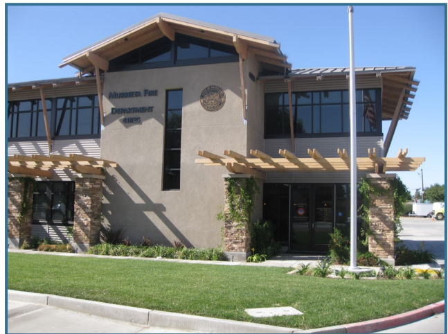
The Murrieta Fire & Rescue is prepared to respond to a variety of emergencies.
