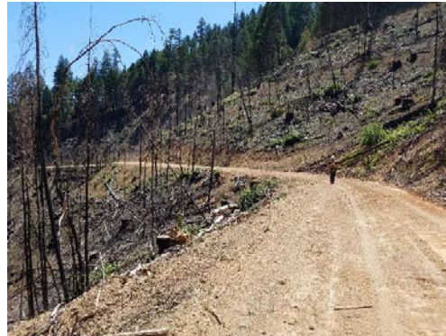
Figure 10: A midslope road on a post-fire Emergency with a road slope of < 5%.
