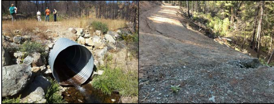
Figure 6: Two crossings, a culvert crossing of a Class II watercourse with a “Trace” discharge (left) and extra rock added on the outboard edge, and a dry ford crossing on a Class III with rill erosion on the eroding road prism (partially shown) and failing outboard edge, with a 15-540 yard 3 discharge estimate.
