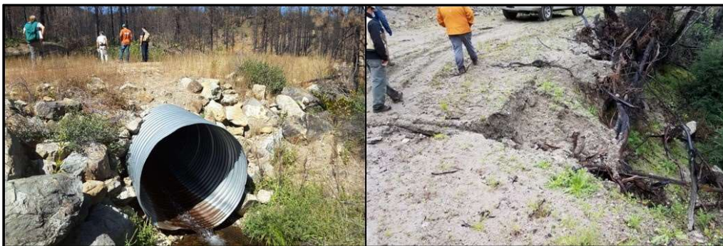
Figure 6: Two crossings, a culvert crossing of a Class II watercourse with a “Trace” discharge (left) and extra rock added on the outboard edge, and a dry ford crossing on a Class III with an eroding road prism (partially shown) and failing outboard edge, with a 5-10 yard 3 discharge estimate.
