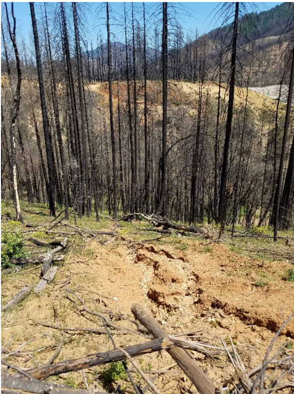
Figure 11: Gully erosion below a skid trail waterbar, cause in part by accumulated upslope drainage, which discharged to a watercourse.
