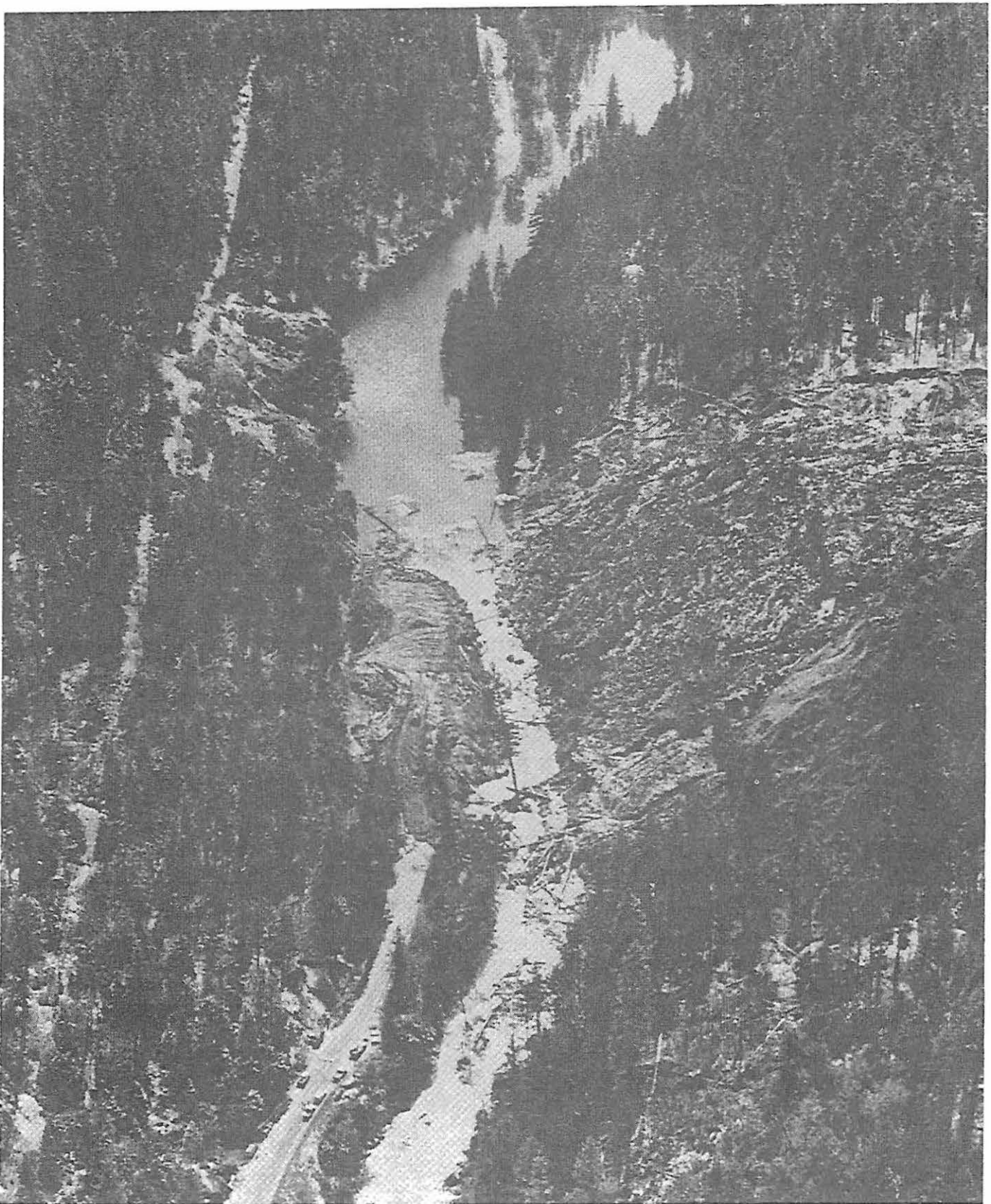
The U. S. Highway 50 landslide (right) looking east. A harvesting plan for the timber on the slope was submitted in 1988. Photo courtesy of Cal Trans.
