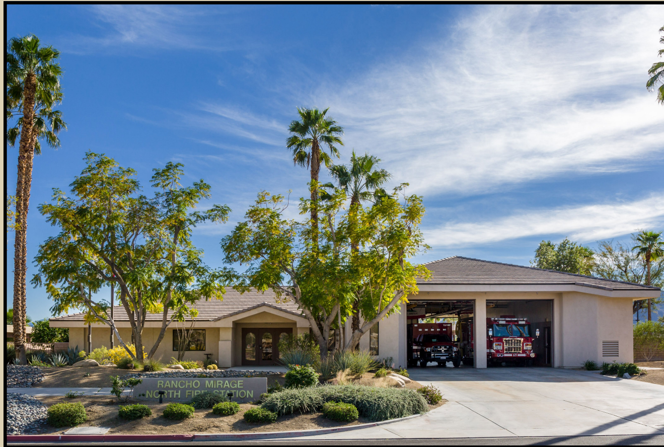
Rancho Mirage Fire Station 69.
